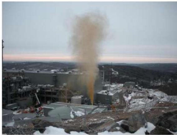
Figure 3. The cleaning of fuel gas piping at the Kleen Energy site on January 30, 2010, one week prior to the incident; a “gas blow” method was used to remove debris from the piping. The brown cloud seen here is indicative of debris being blown from the line.
