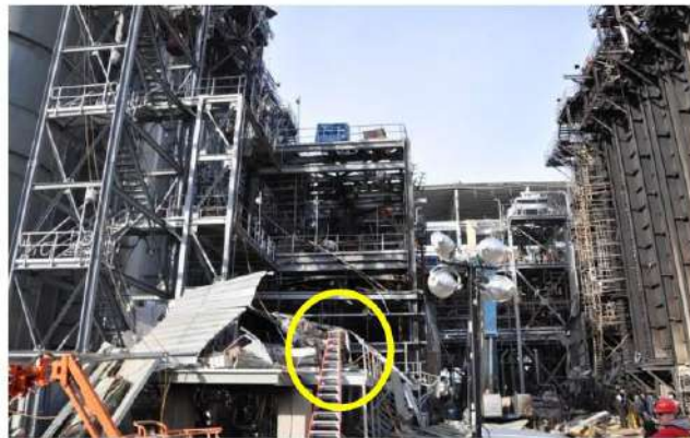
Figure 1. The general location of open-ended pipe where natural gas was vented to the outdoors at time of incident (yellow oval). The actual vent piping is obscured by the structure and scaffolding.
